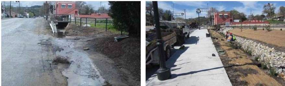
21 st Street looking east before (left) and after (right) redesign
