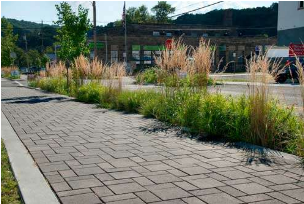
Permeable pavers and bioswales improve stormwater management.
