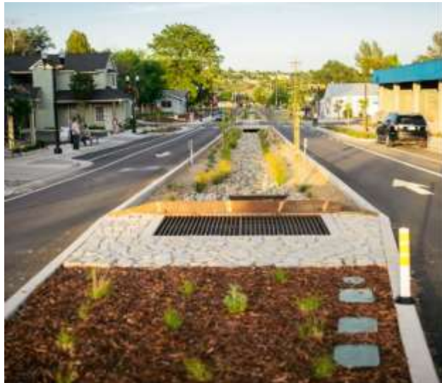
Open median channel in the center of 21 st Street
